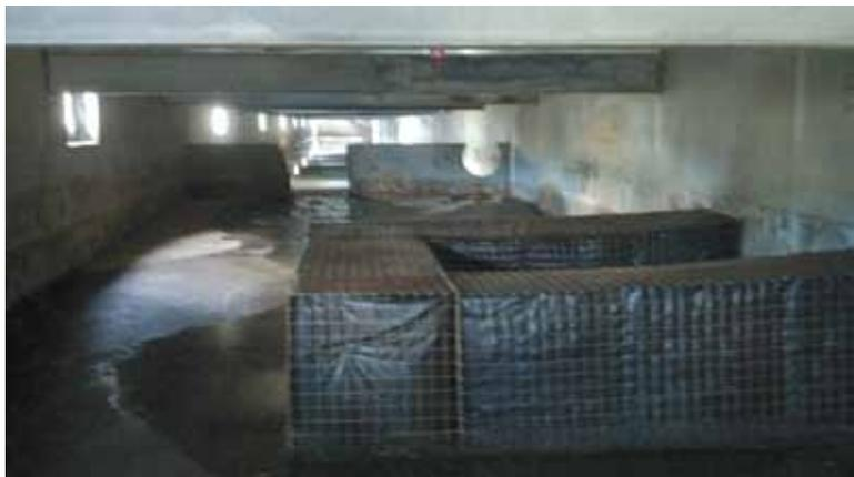
Vault design with only one catch basin being active and protected by the BFG. The other 5 have been closed off.
